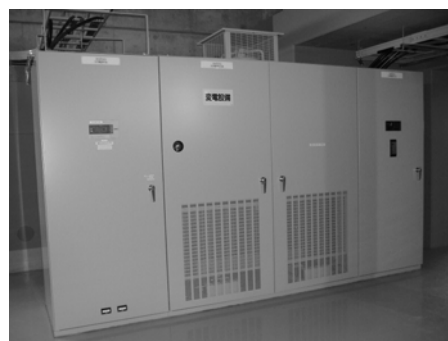
Fig. 2 MV switchgear.
