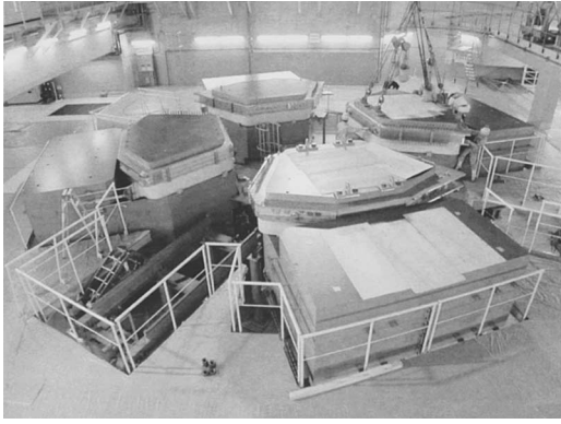
Fig. 3. Photograph of the IRC vault that was taken in November 2003. The lower parts have been assembled for all the four sector magnets.
