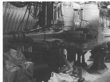
Fig. 1. RHIC pC CNI polarimeter installed in RHIC.
