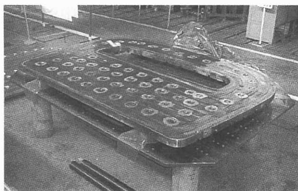
Fig. 2. The proto-trim-coil vessel after the closing weld. The numerous circular marks indicate the stay-rod welds.
